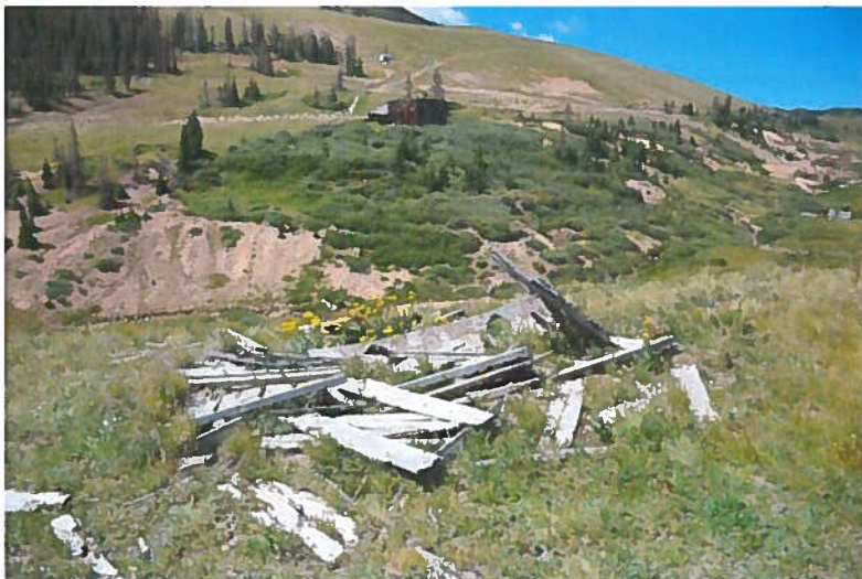
Figure 10, Building # 3, Two Door Privy, looking south
