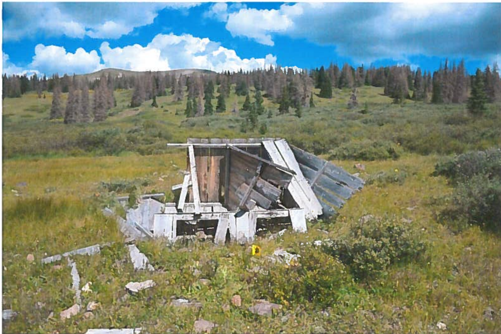
Figure 38, Building #28, Collapsed 2 hole/2 door Privy. Looking north.
