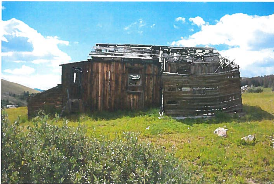
Figure 30, Building #20, looking west.
