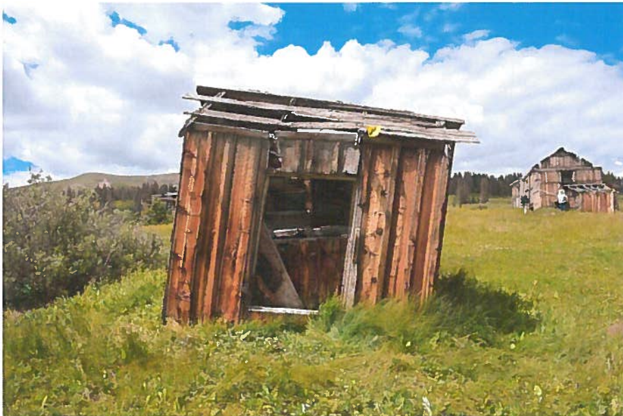
Figure 24, Building #14, looking north.
