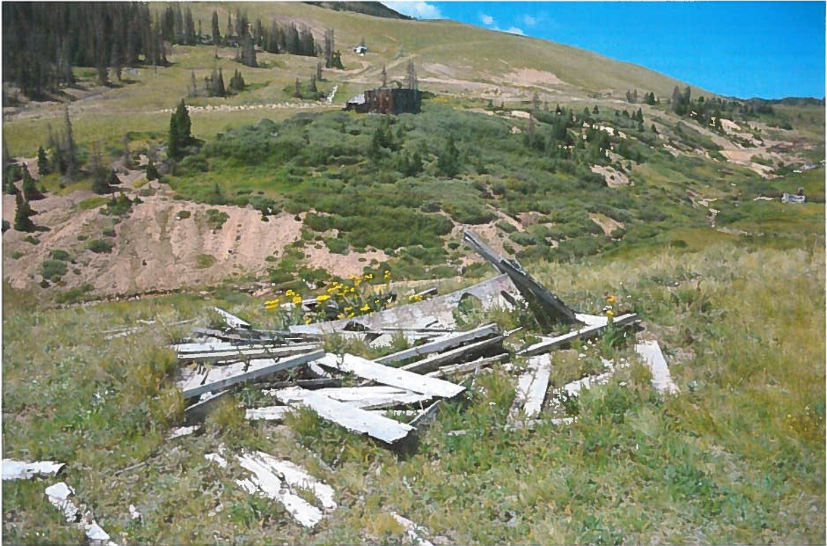
Figure 13, Building # 3, Two Door Privy, looking south.
