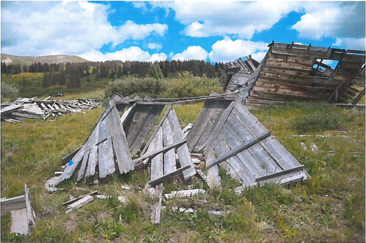
Figure 18, Building #8, Two Door Privy, looking north
