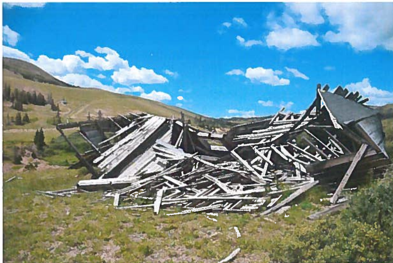
Figure 19, Building #9, large collapsed building, looking southwest.
