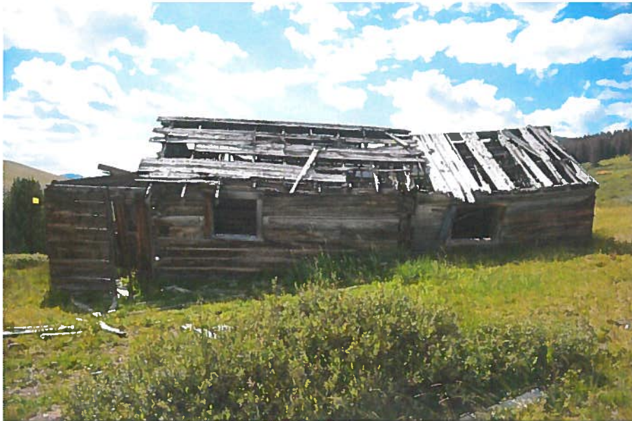
Figure 32, Building #22, looking west.
