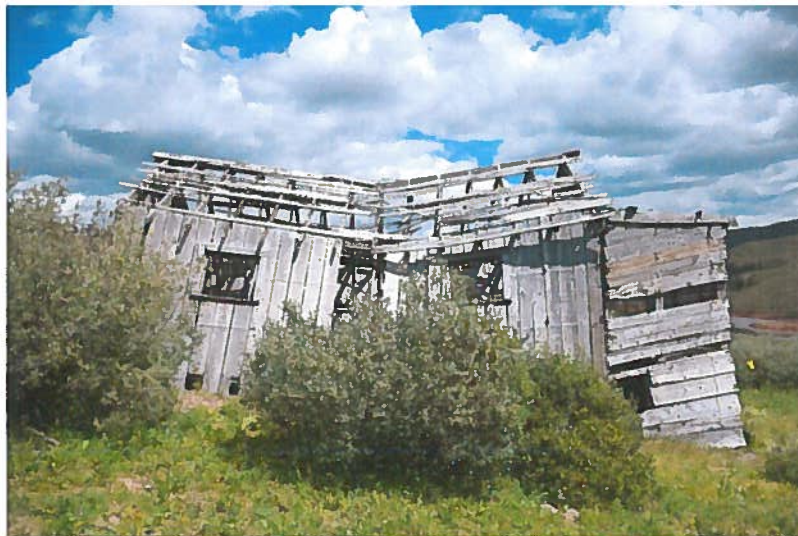
Figure 23, Building #13, looking east.
