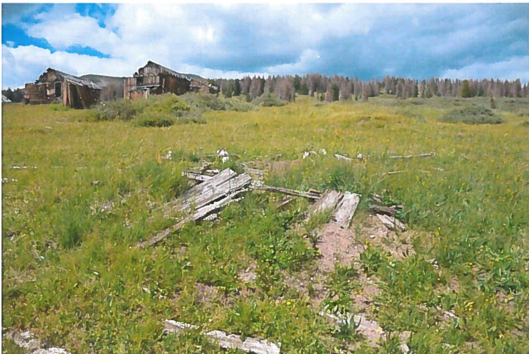
Figure 26, Building #16, collapsed structure, possible Hydrant, looking north.
