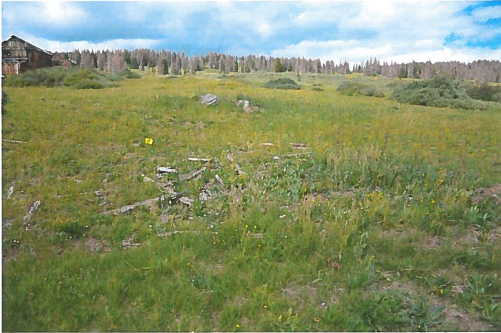
Figure 27, Building #17, Collapsed, function unknown. Looking north.
