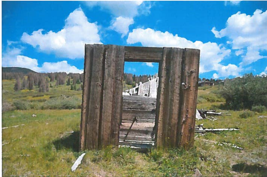
Figure 14, Building #4, Water Hydrant, looking north
