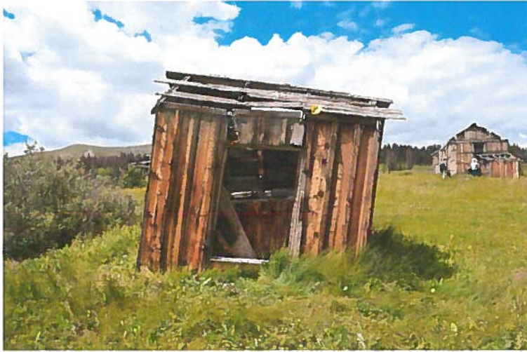
Figure 9, Building 14 Hydrant Pump House
