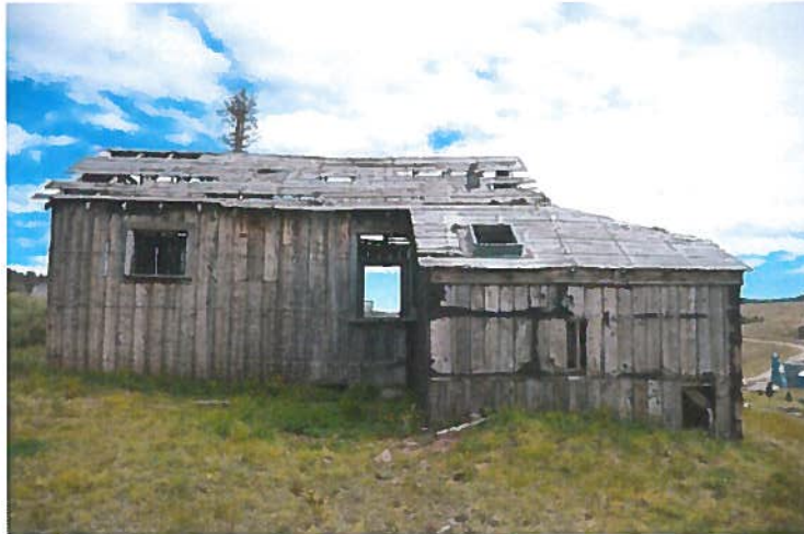
Figure 12, Building #2, looking east
