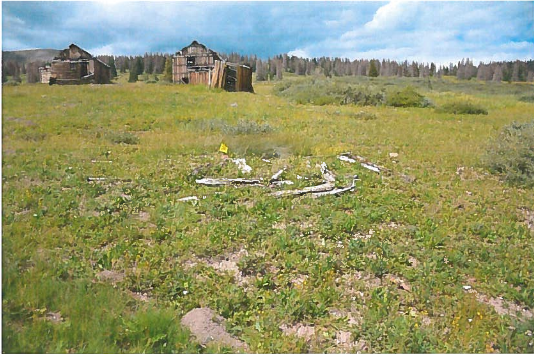
Figure 25, Building #15. Collapsed structure, possible Privy, looking north.
