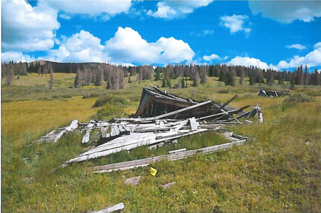
Figure 35, Building #25, collapsed residential structure, 17' x 12'. Lean-to addition on north end, 13'6" x 9'. Looking north.
