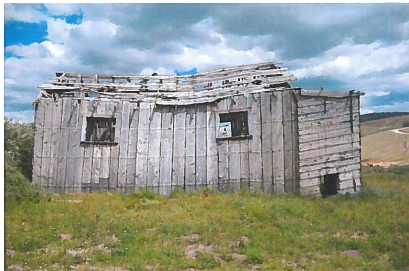
Figure 22, Building #12, looking east.
