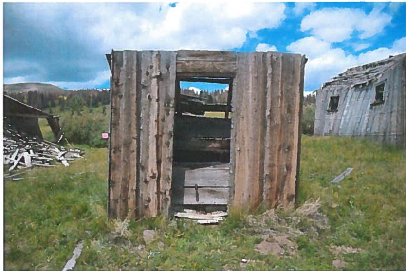
Figure 20, Building #10, Water Hydrant, facing north.
