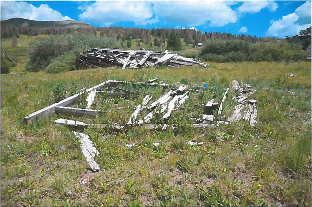
Figure 16, Building #6, looking north
