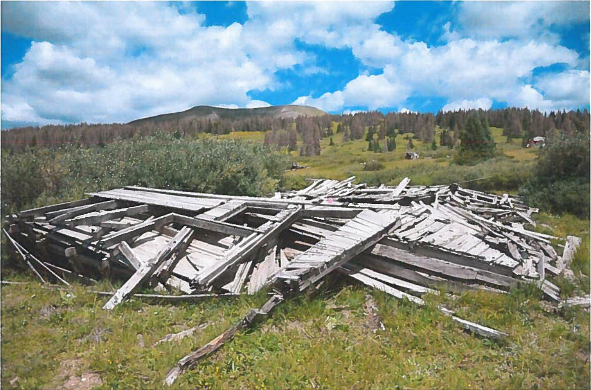
Figure 17, Building #7, looking north
