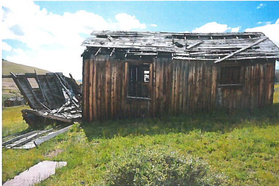
Figure 31, Building #21, looking west.
