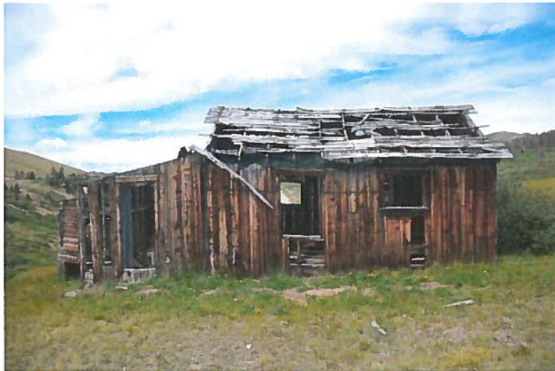
Figure 11, Building #1, looking west
