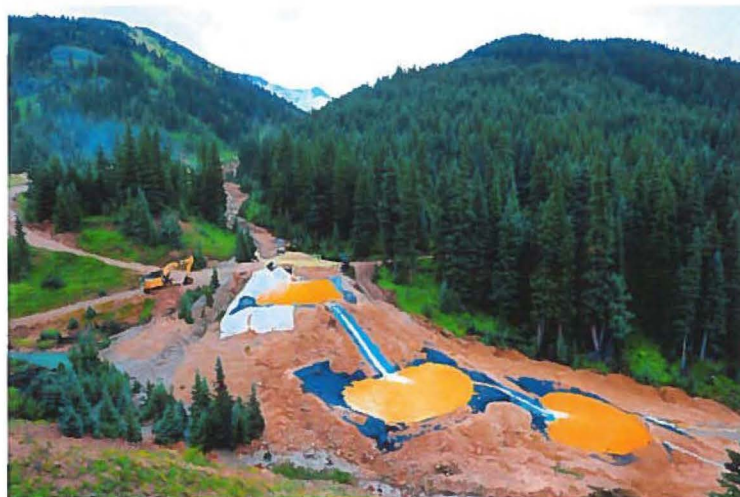
Figure 6: Settling Ponds used to process the Gold King Mine Waste, Data from The Albuquerque Journal , accessed June 15, 2016, http://www.abqjournal.com/628976/gold-king-mine-spill-a-disaster-waiting-to-happen.html
