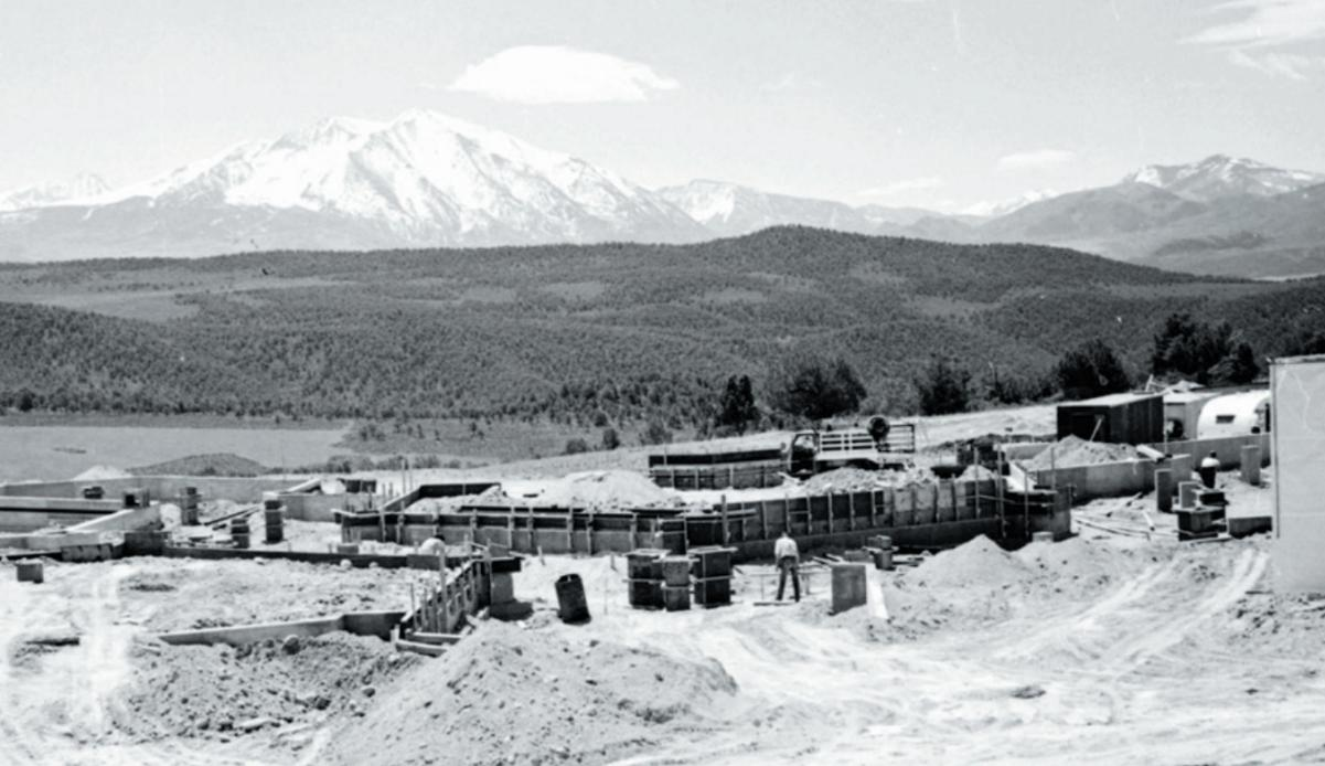
Foundation construction at West Campus near Glenwood Springs prepared the site for prefabricated modular buildings, transported from Denver, and identical to those installed at East Campus in Leadville.
