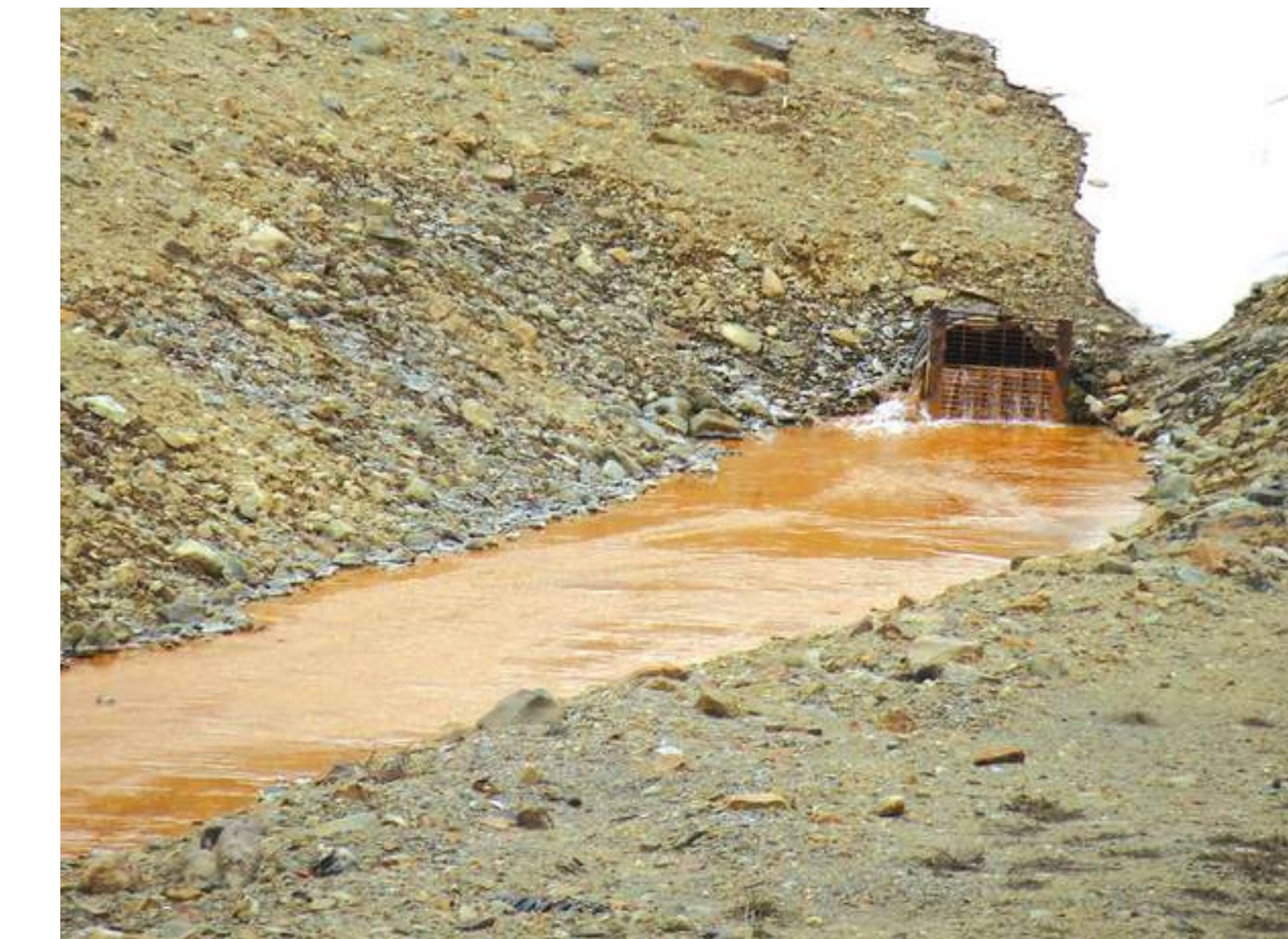
Tainted water in the American tunnel at Gladstone pours into the portal at Cement Creek in 2012
