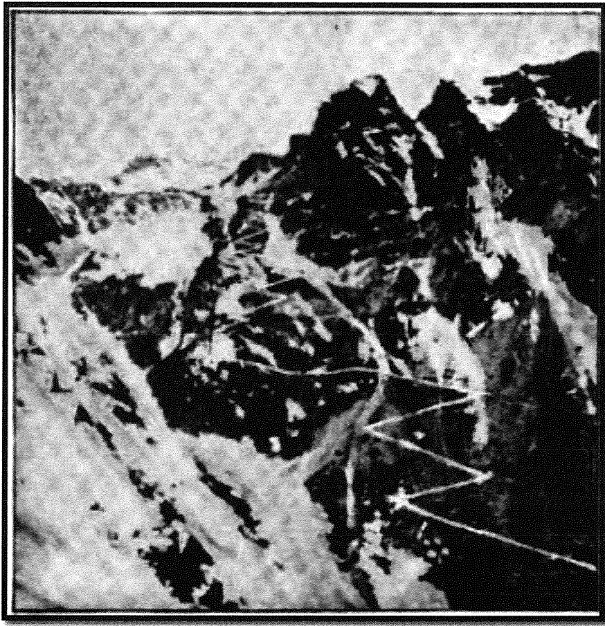
Fig. 4: Switchbacks to Silver Lake Reprinted from, Western Electrician , August 31, 1895
