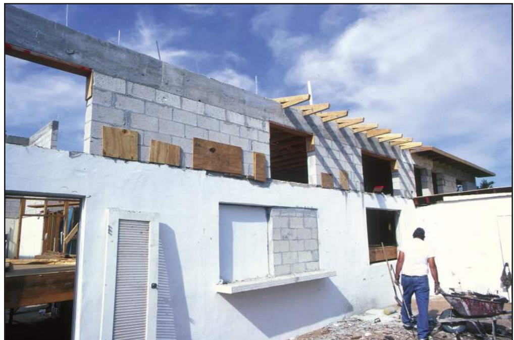
Figure 67 The extended first-story walls.
