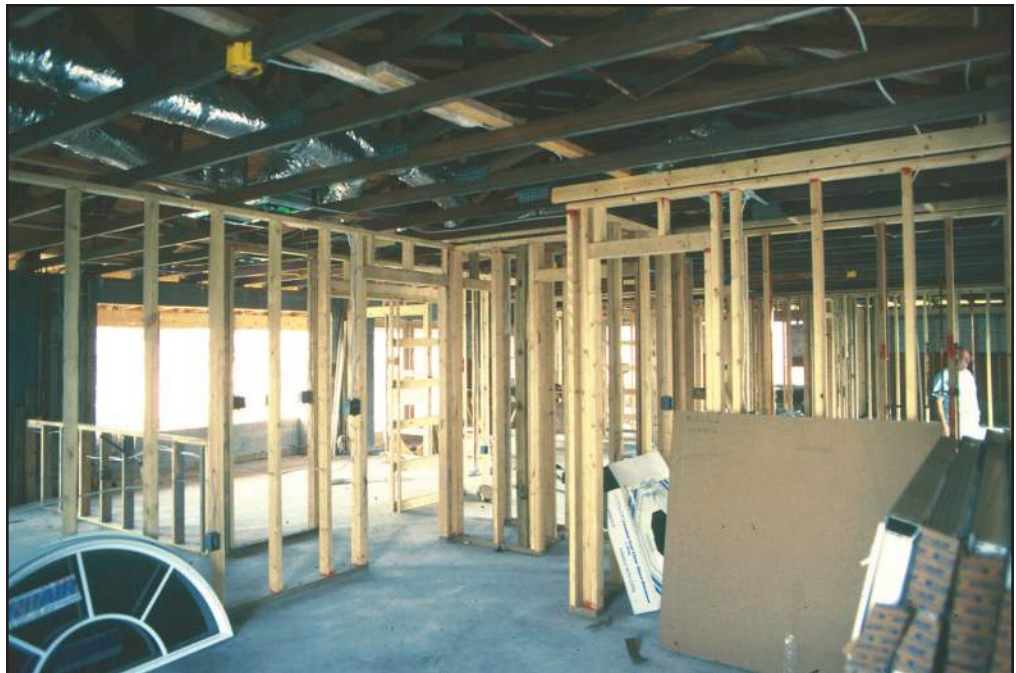
Figure 30 Interior partition walls and utilities are added.
