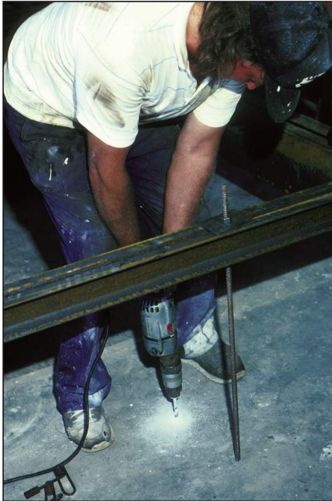
Figure 77 ... install anchors ...
