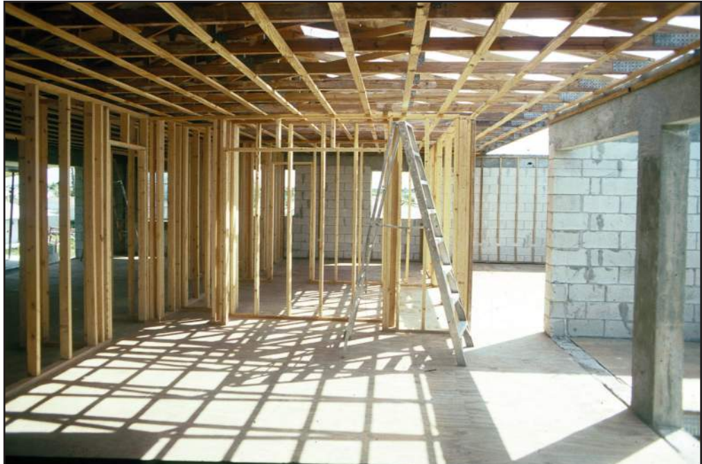
Figure 34 After the new concrete slab is poured, wood framing for interior walls is added.
