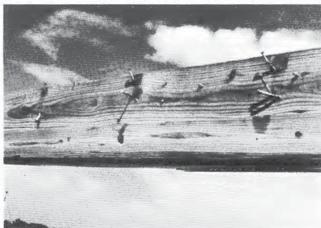
Figure 4.26. Toe Nailing Provides Limited Pull-Out Resistance
