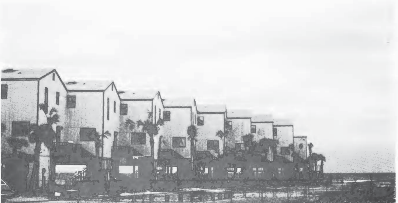
Figure 3.27. This is a good example of how the configuration of a cluster layout can contribute to functional advantage as well as visual appeal. The sawtooth arrangement allows for two sides of each unit to have access/view to the ocean. This form also breaks up the long, continuous (and often monotonous) wall approach, thus adding variety and interest. With this configuration the materials, treatment and form of the units can be simple but still attractive.
