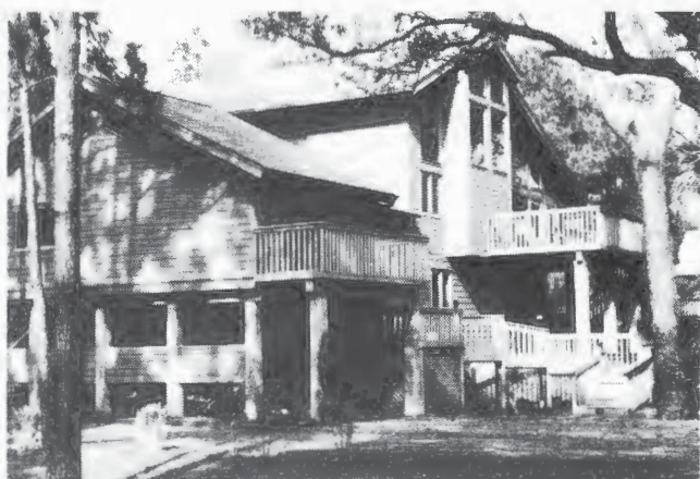
Figure 4.3. Elevation by Posts
