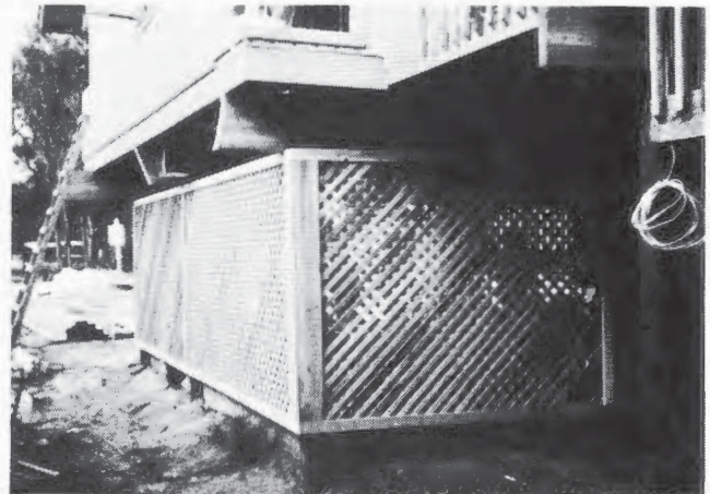
Figure 4.54. Breakaway Walls
