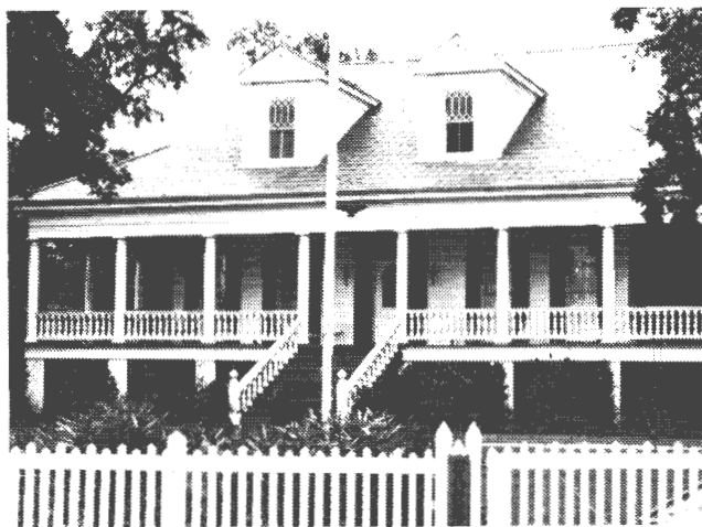
Figure 4.15. Pier Foundations
