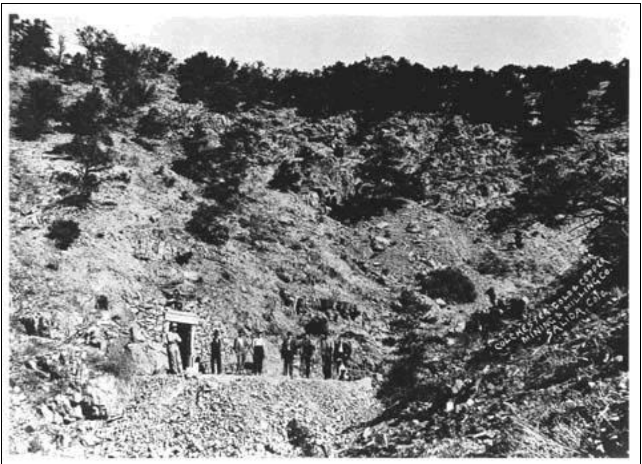
Tunnel No. 2, Colchester Gold & Copper Mining & Milling Co. in Salida in 1890
