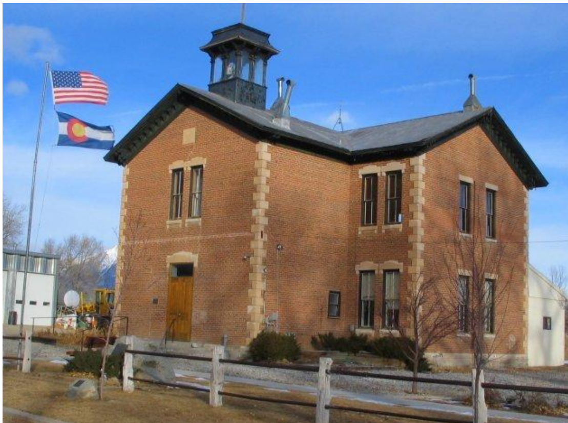
The old brick Schoolhouse which today is utilized as the City Hall Building
