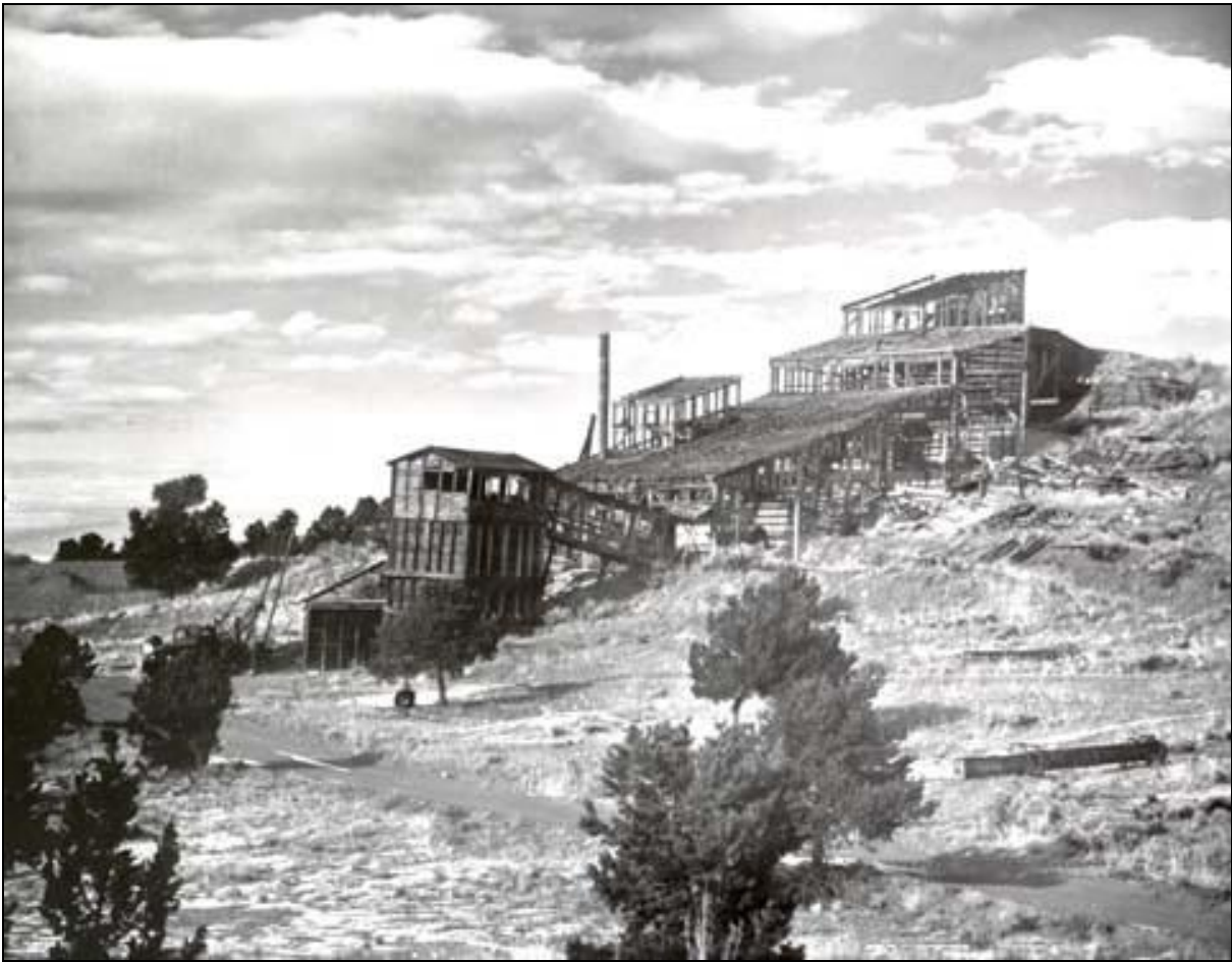
An old inactive silver mine in Salida (photo by J. Todd: Salida Library )
